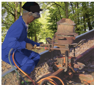
Figure 3.11 Thermit process for joining railway tracks
